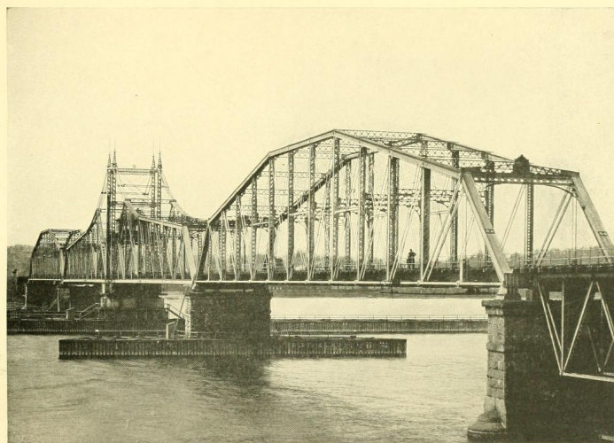
RAILROAD BRIDGE OVER THE THAMES From Winthrop Neck to Groton stretches the Thames River Bridge, one of the greatest engineering feats of the century, 1,423 feet long with a 503-foot draw, and the longest double track drawbridge in the world. It is proportioned for a moving load of two 80-ton locomotives followed by a train load 3,000 pounds per foot.
